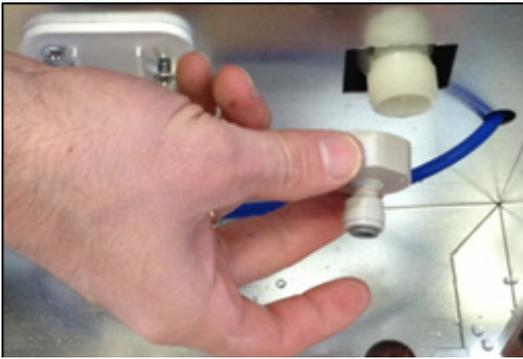
The blue pipe connects to the grey fitting which can be found underneath the appliance. The grey fitting can be unscrewed, and the blue pipe slots into it. Then screws back onto the appliance.
