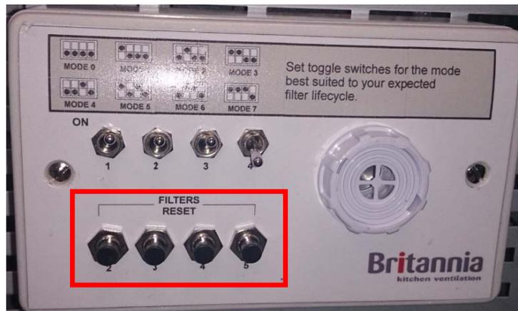
**Filter Stage Reset Panel - FILTERS RESET**
