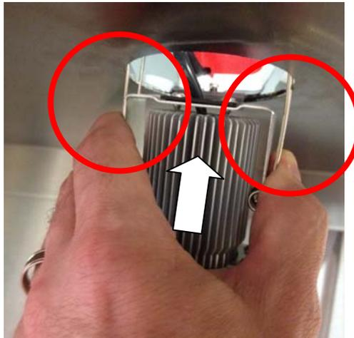
**Squeezing the Clips to Replace the Lamp to the Canopy**
