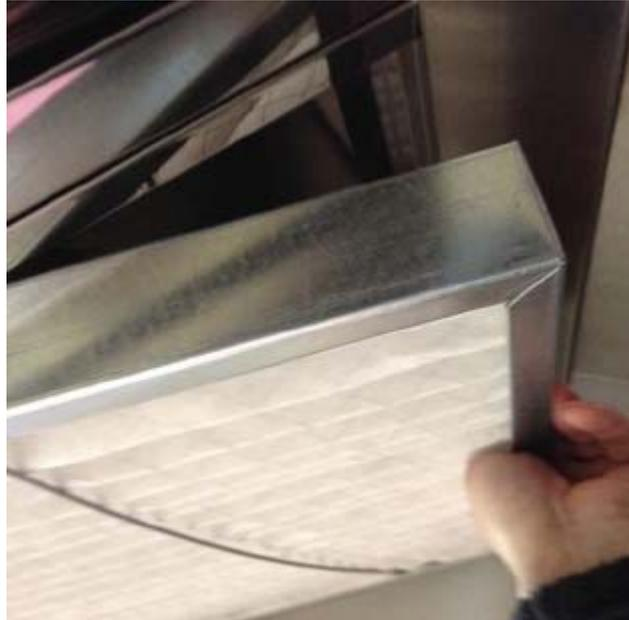
***Removing the Stage 2 filter***
