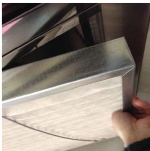
**Removing the Stage 2 filter**
