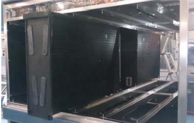
***Removing Each of the Stage 5 Carbon Cells***
