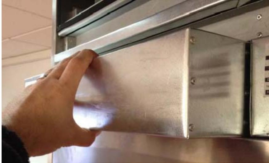
***Sliding the Stage 3 Filter Panel Forward***
