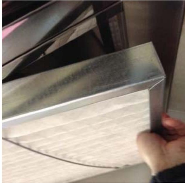
***Replacing the Stage 2 Filter Panel***
