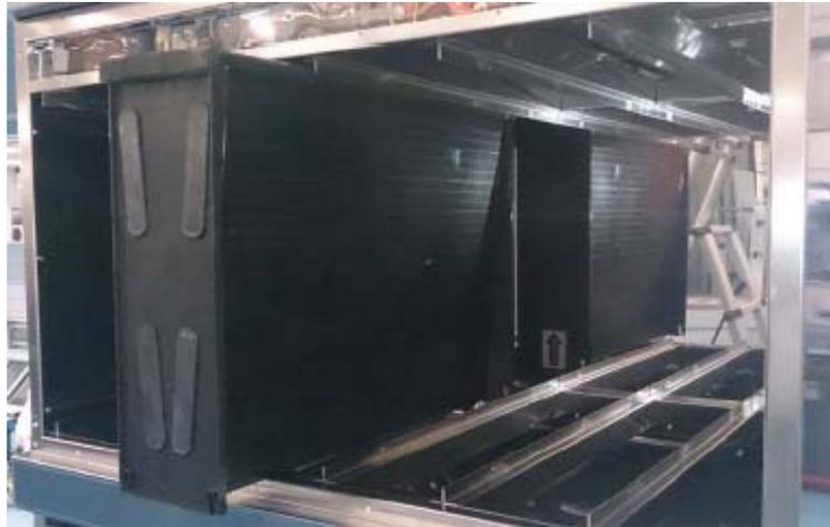
***Replacing Each of the Stage 5 Carbon Cells***
