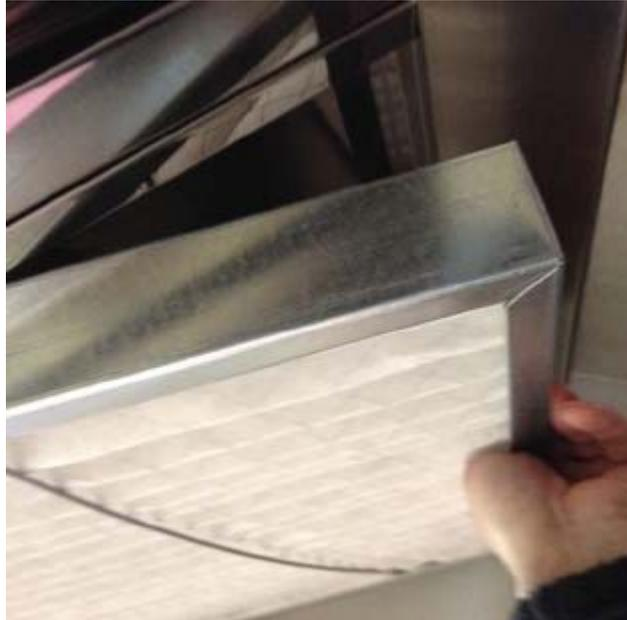
***Removing the Stage 2 filter***
