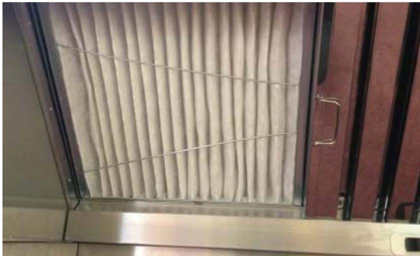
***Stage 2 Filter Panel Replaced***
