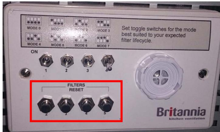
**Filter Stage Reset Panel - FILTERS RESET**
