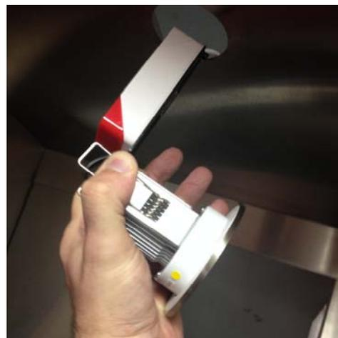
**Removing the Fitting from the Canopy**
