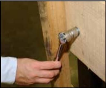
Removing skid from bottom of cabinet.
