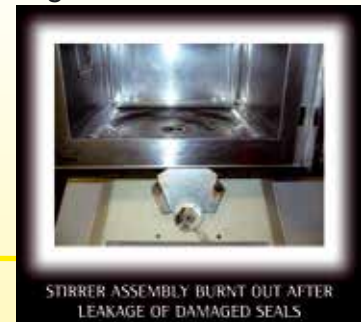
Damaged seals on the ceramic base
